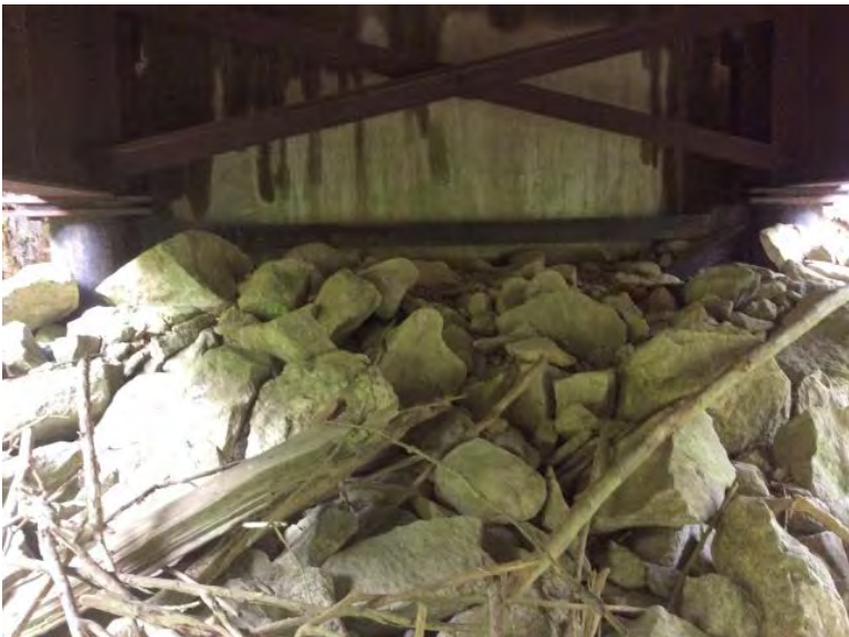
Left Bank Abutment when facing downstream
