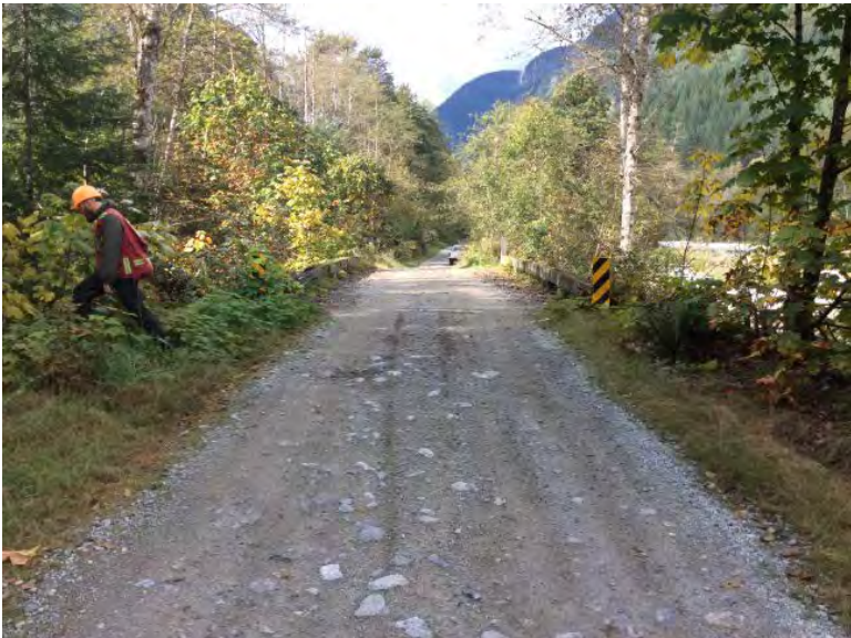
Approach from Right Bank when facing downstream
