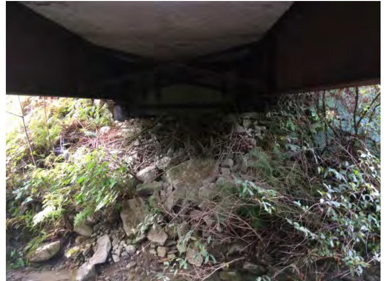
Right Bank Abutment when facing downstream
